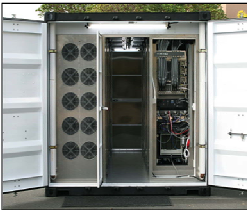
Figure 5. Sun Microsystems modular data center.
