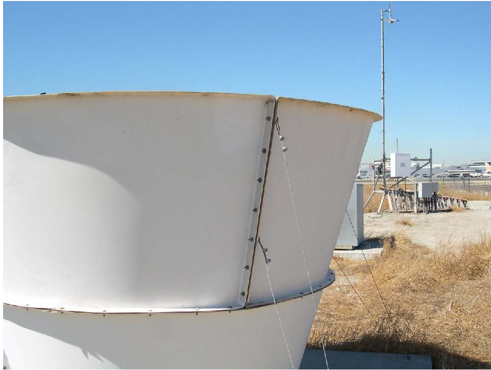
Figure 3. Sensor field site equipment. Foreground is sodar baffle anchored to cement pad. Background shows tower with mounted sensors. Electronics box is seen at base of tower.
