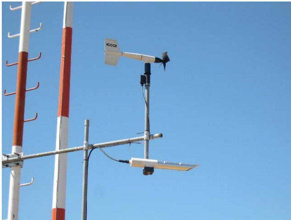
Figure 6. Propeller and vane anemometer system mounted atop tower.
