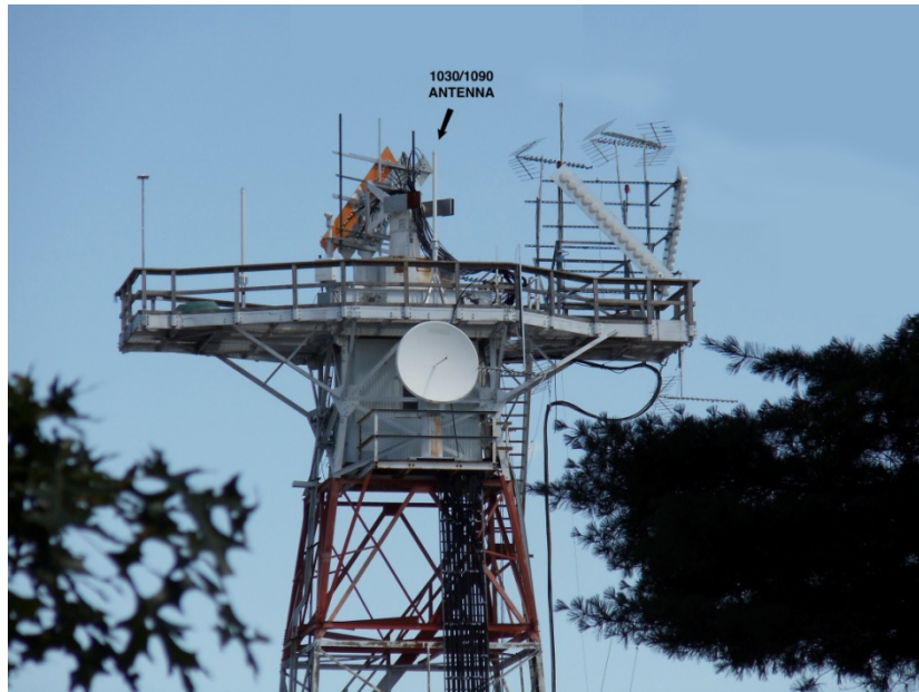
Figure 5. Tower with antennas
