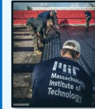
Solar sys. installation
