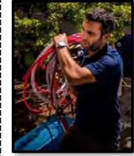
Water sys. installation
