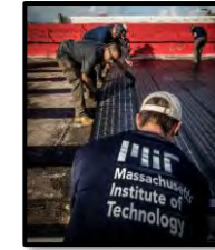
Solar sys. installation
