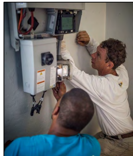
Installing the off-grid solar inverter
