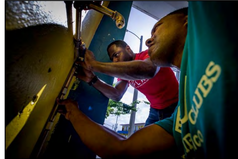
Taps installed at front of Loíza Club
