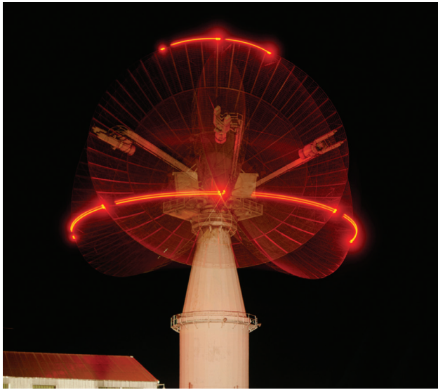
FIGURE 1. The original 1957 Millstone Hill radar that detected Sputnik I was upgraded in 1962 from an ultrahigh-frequency radar operating at about 450 MHz to an L-band radar operating at 1.295 GHz; the new antenna installed during this upgrade is pictured above. Millstone provides 18,000 deep-space satellite observations a year, making it a key contributor to the national deep-space surveillance program.
