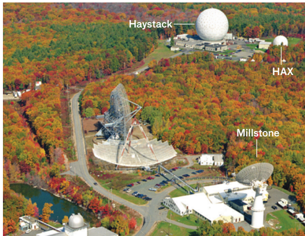
FIGURE 4. The Lincoln Space Surveillance Complex, located in Westford, Massachusetts, comprises three major radars—the Millstone Deep-Space Tracking Radar (L band), the Haystack Ultrawideband Satellite Imaging Radar (X and W band), and the Haystack Auxiliary (HAX) Radar (Ku band). The complex provides key data for space situational awareness and valuable information for radio astronomy.
