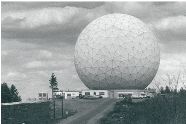
FIGURE 3. The construction of Haystack, seen from its exterior in the photograph above, was completed in 1964.
