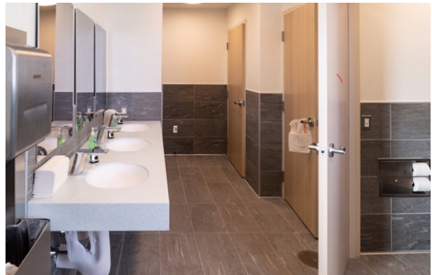
Bathroom after renovation.
